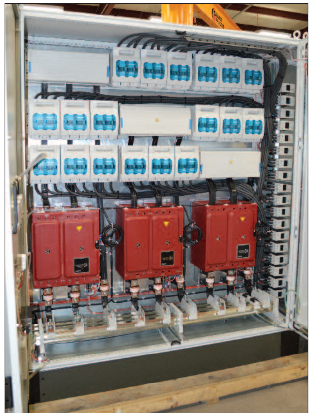
cUL 3200A SCR panel with buss bar
