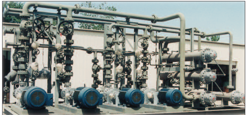
Dual zone, mag drive pump for petrochemical
